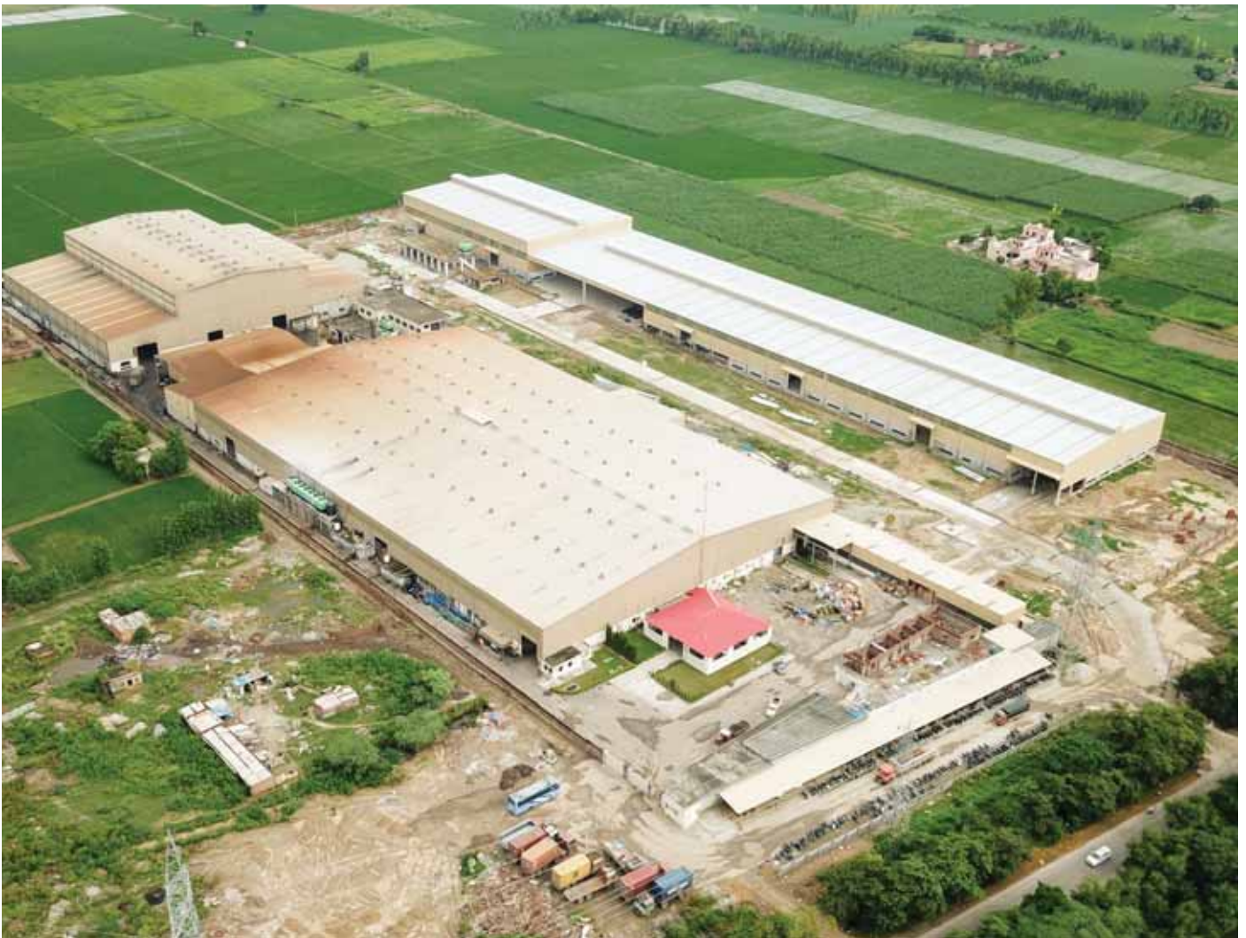
Bird's Eye view of the existing and new SUV shed in Unit II of the Company
